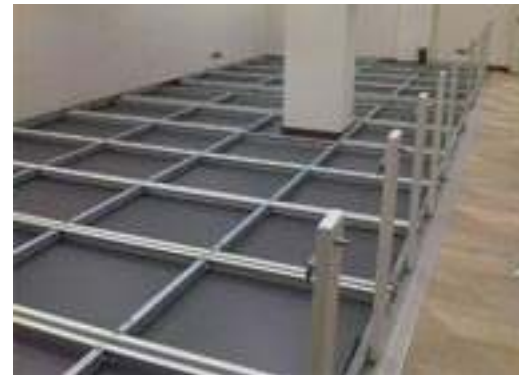
Laying out the floor and rail framework for the mobile system.
